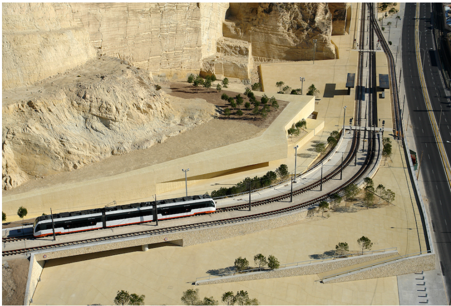
Figure 1: Flyover and retaining walls in Sangueta station, Alicante metropolitan railway.
