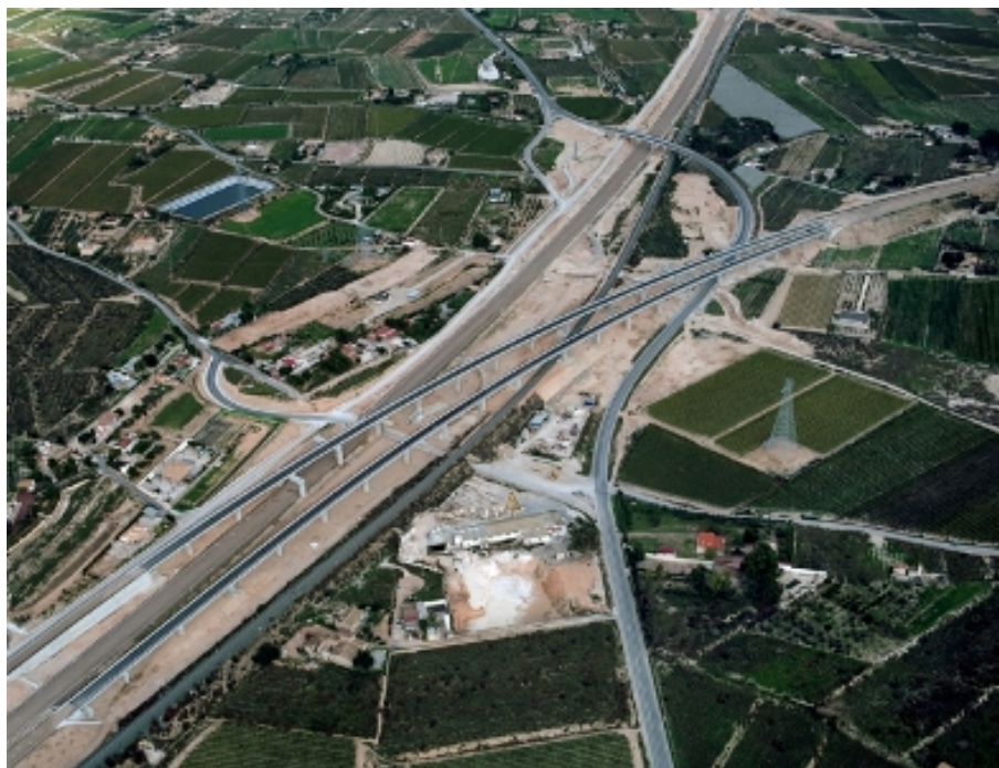
Figure 2: Viaducts Madrid-Levante high speed railway in Novelda
