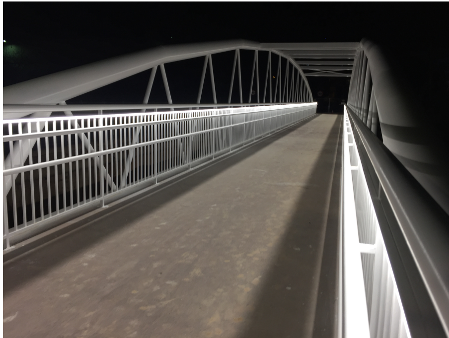
Figure 5: Pedestrian bridge in Villamarchante (Valencia).
