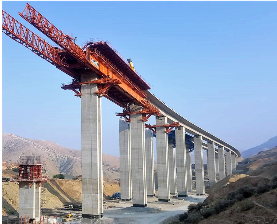
Figure 3: Viaduct 03B during construction (Mascara, Algeria).
