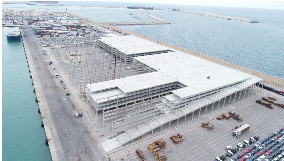
Figure 4: Storage cars building in the port of Valencia.
